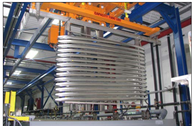
Figure 2. The anodizing line processes extrusions and other complex components, such as luggage racks installed on the roofs of cars.
